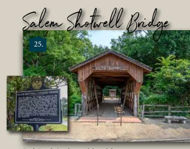
**Park Road:** Southeast Alabama's last surviving covered bridge was originally built by Otto Puls over Wacoochee Creek. Town's lattice truss design, longleaf heart pine, white oak pegs and cedar shakes were used to build the 75-foot-long bridge. (Circa 1900)
